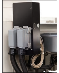
Quick change heater disconnects
